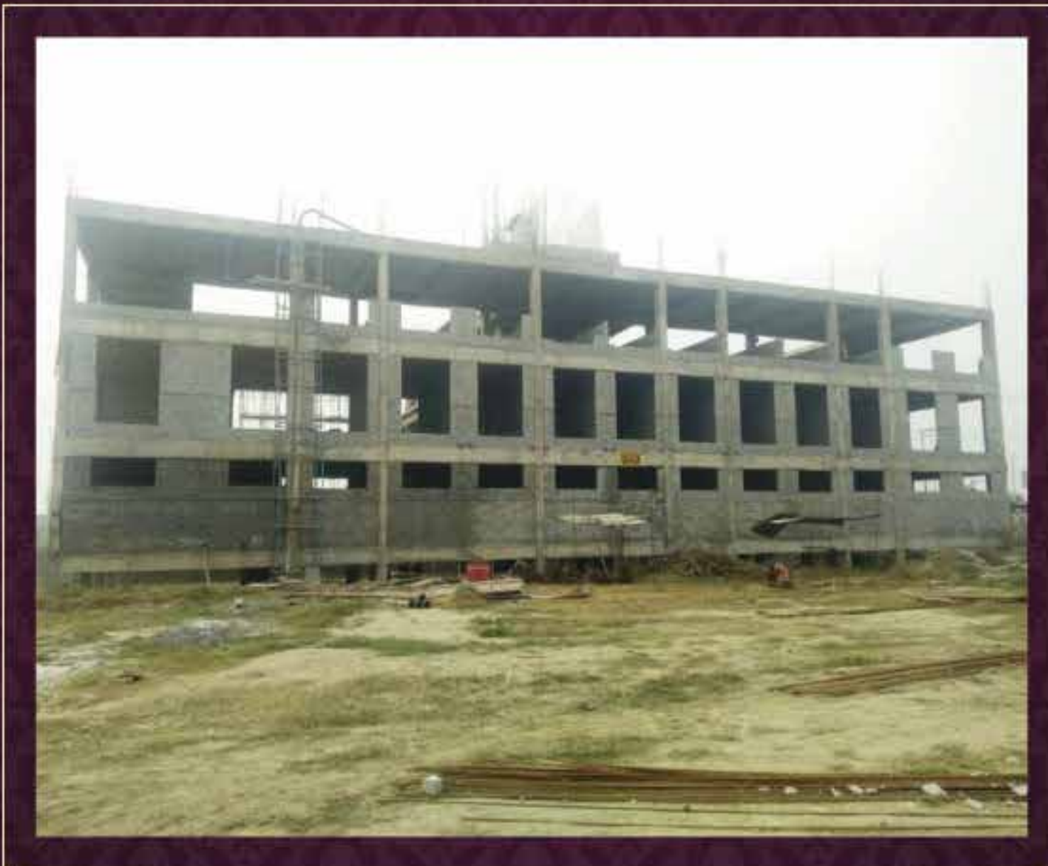
BRICK & PLASTER WORK IN PROGRESS
