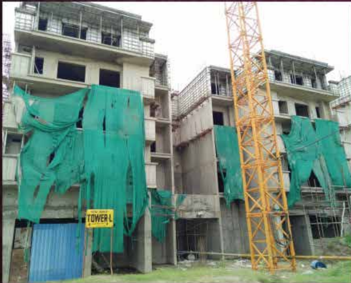
2 ND FLOOR COMPLETED
