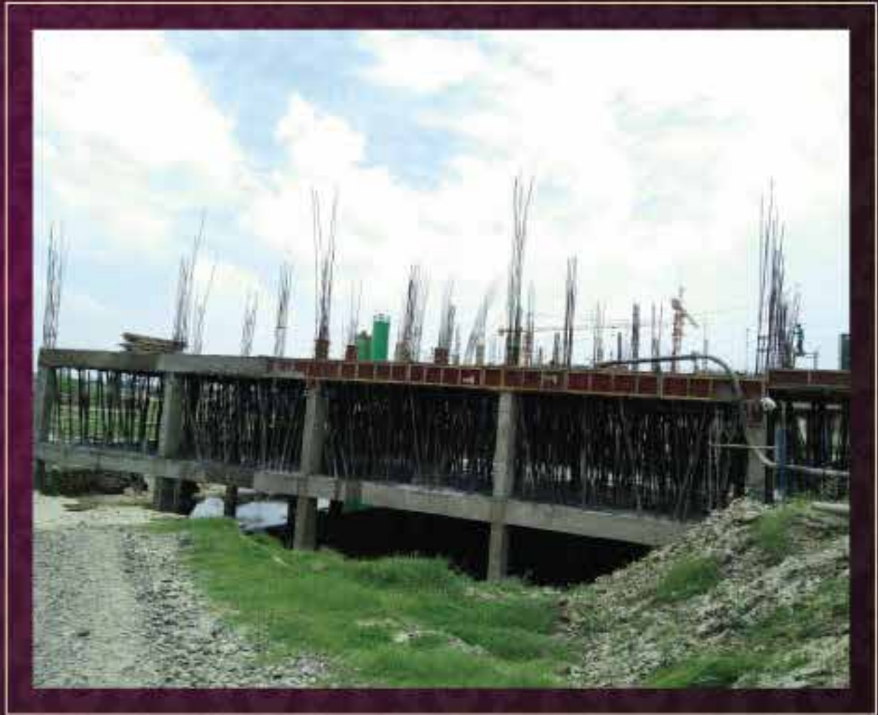
LOWER GROUND FLOOR COMPLETED
