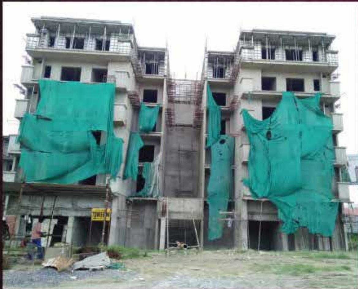
3 RD FLOOR COMPLETED
