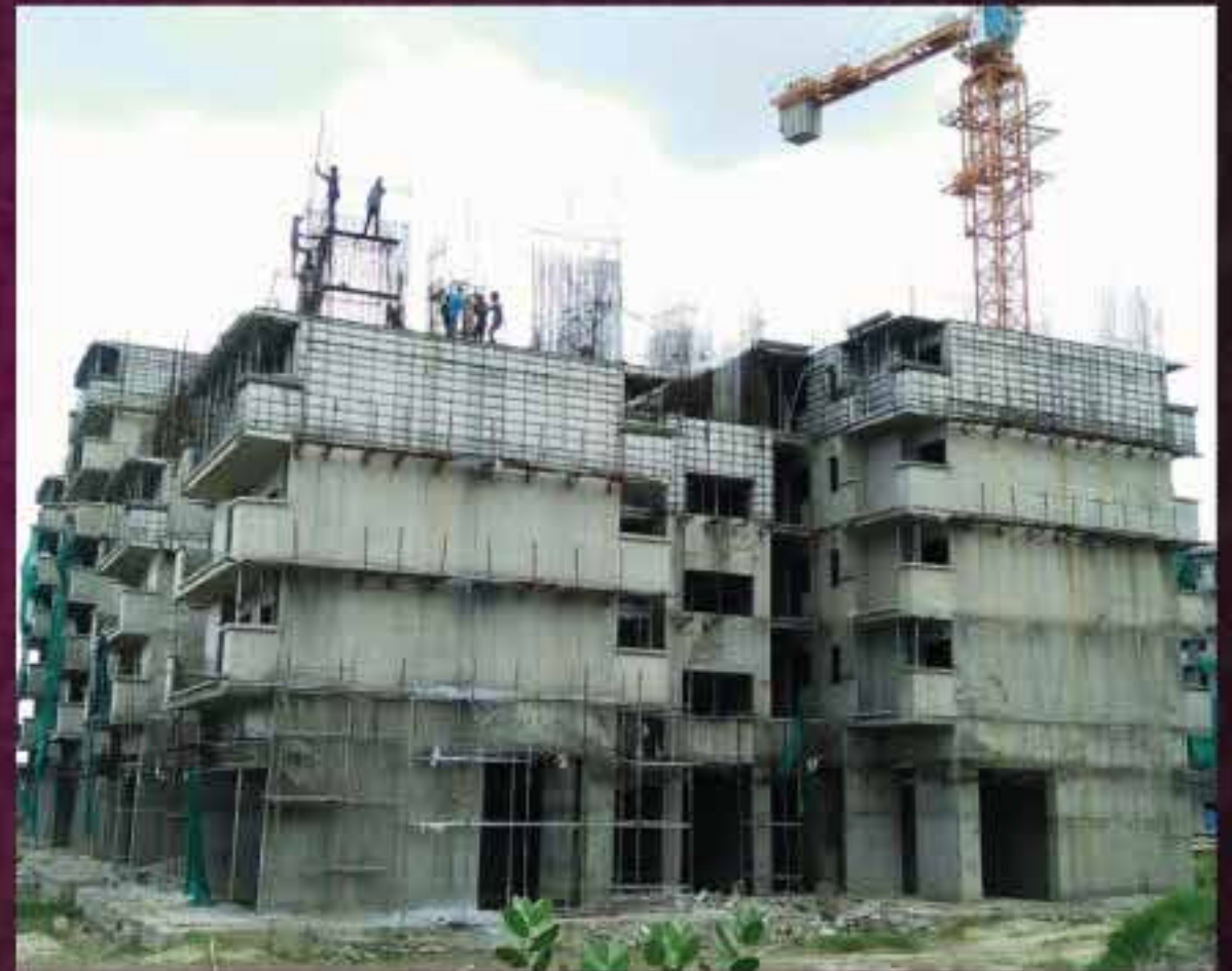
2 ND FLOOR COMPLETED
