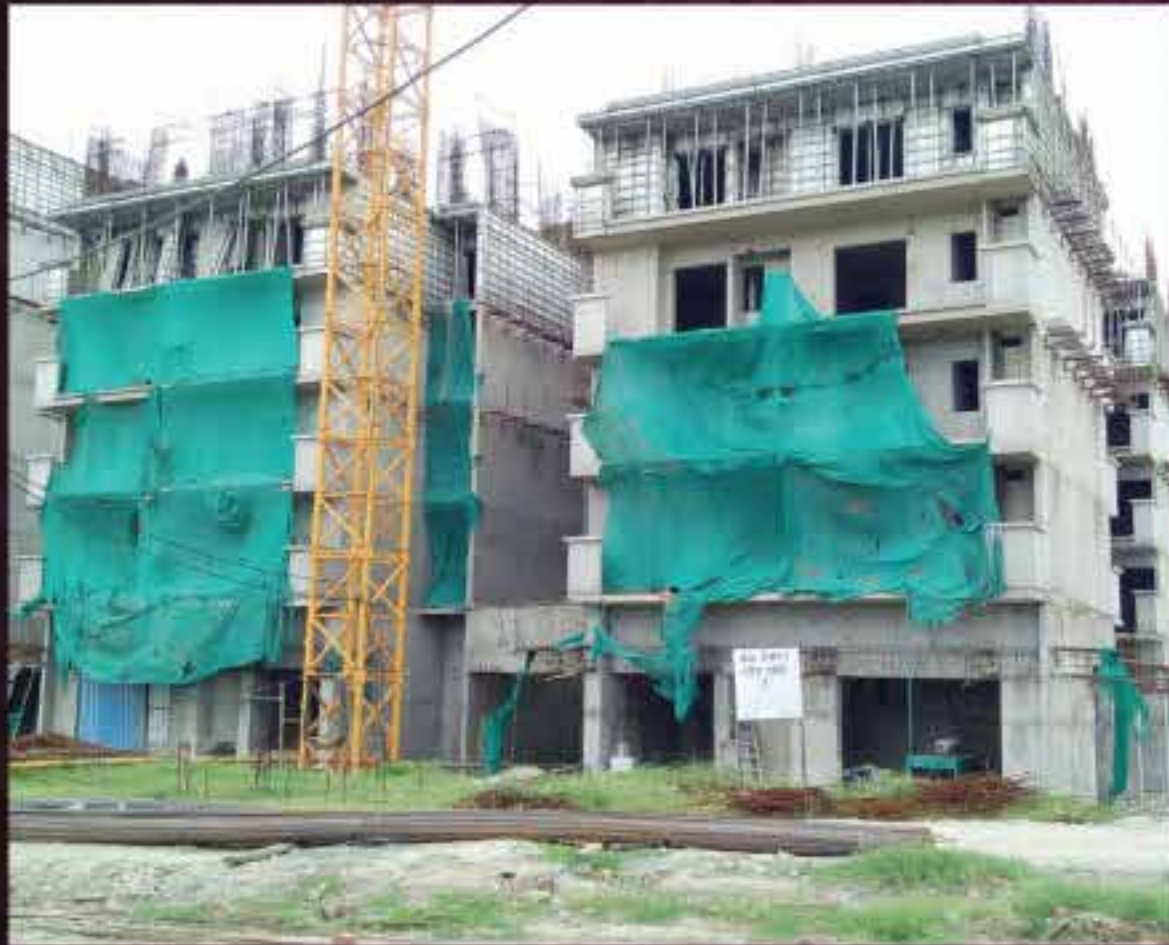
3 RD FLOOR COMPLETED
