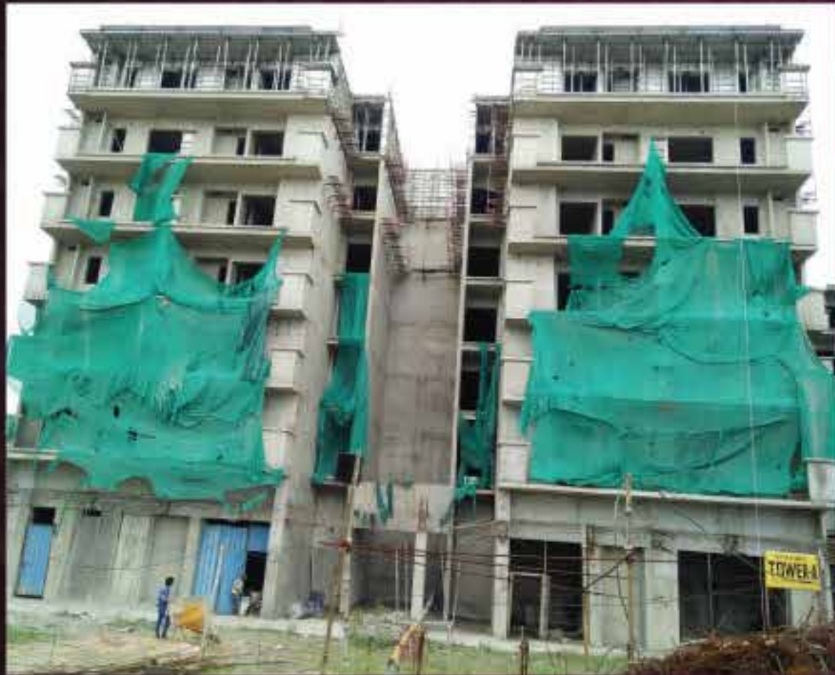
4 TH FLOOR COMPLETED
