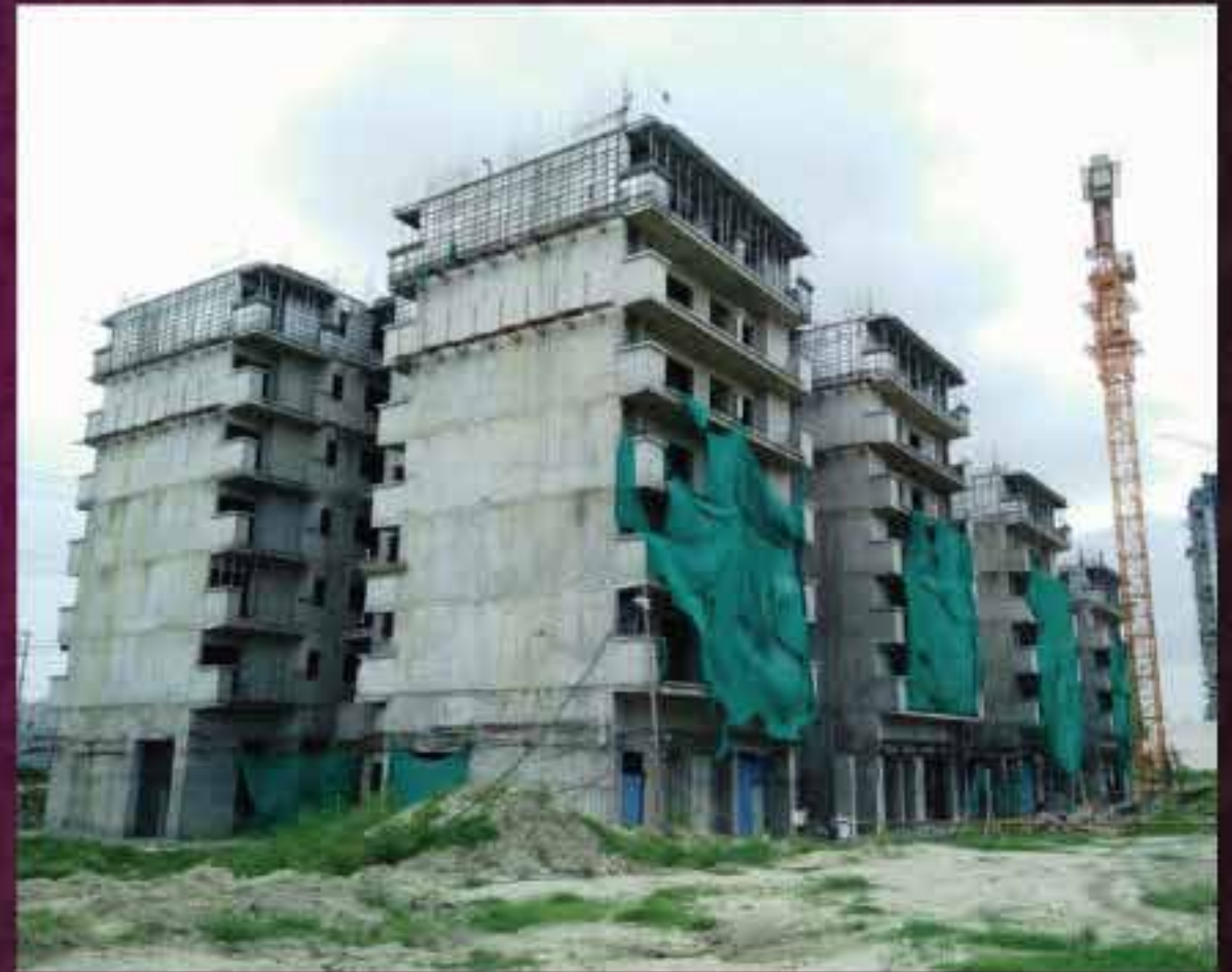
4 TH FLOOR COMPLETED
