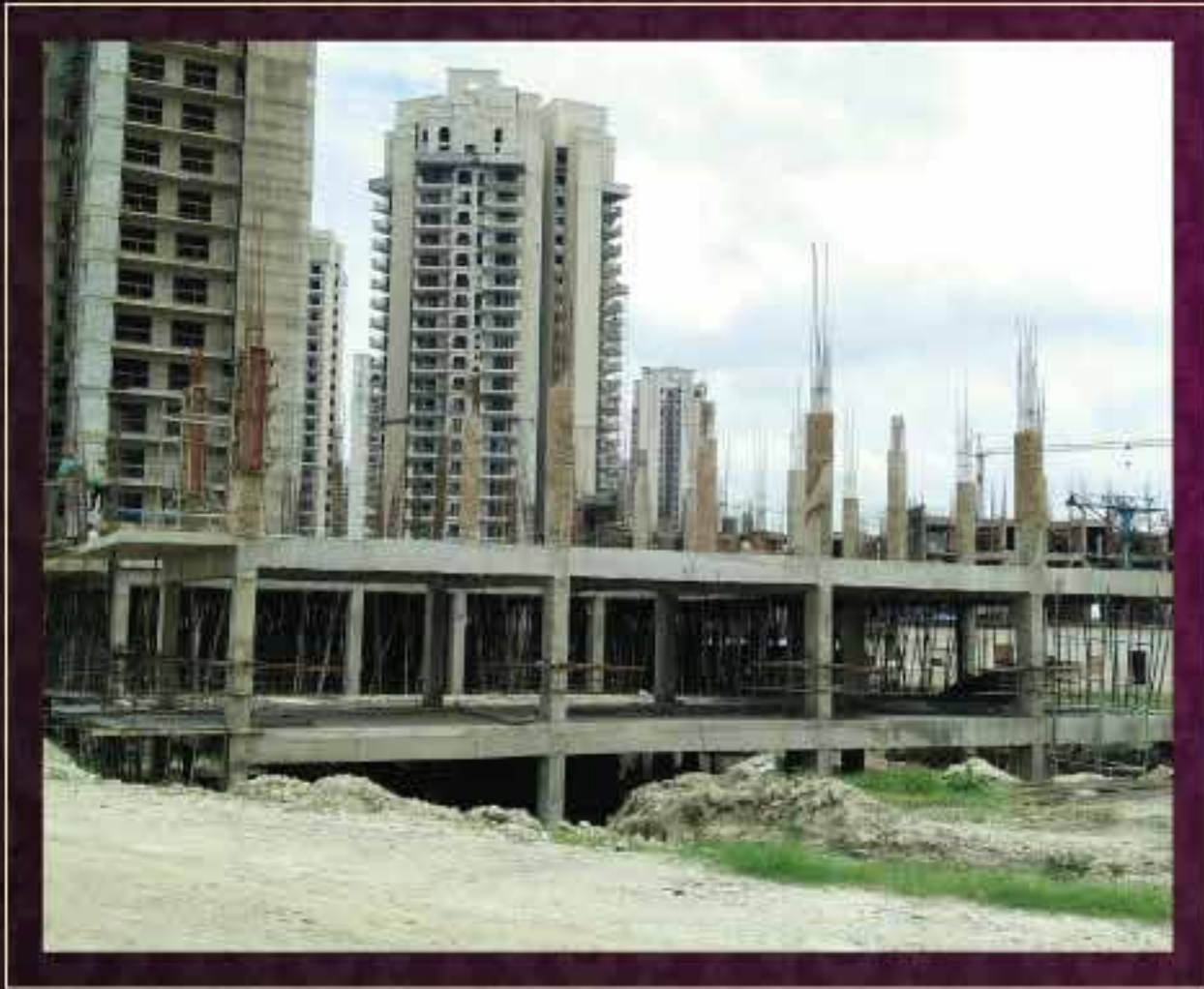
LOWER GROUND FLOOR COMPLETED
