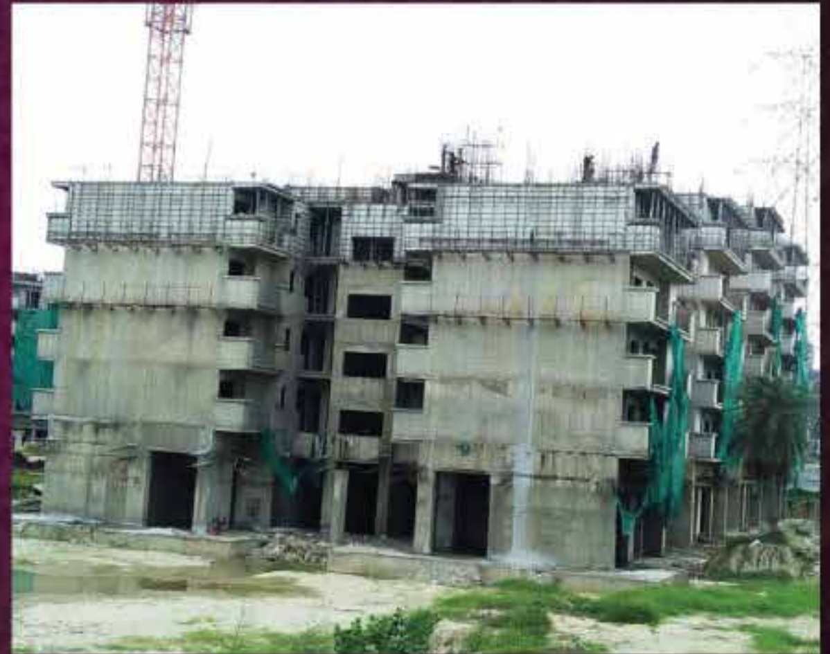
3 RD FLOOR COMPLETED
