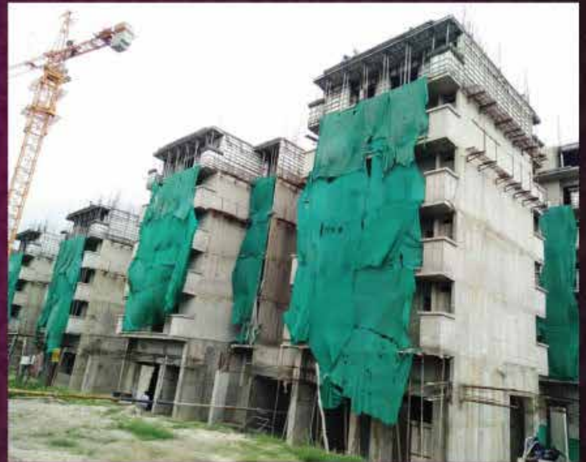
3 RD FLOOR COMPLETED
